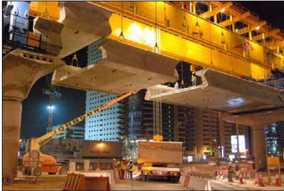
Direct lifting of segments
