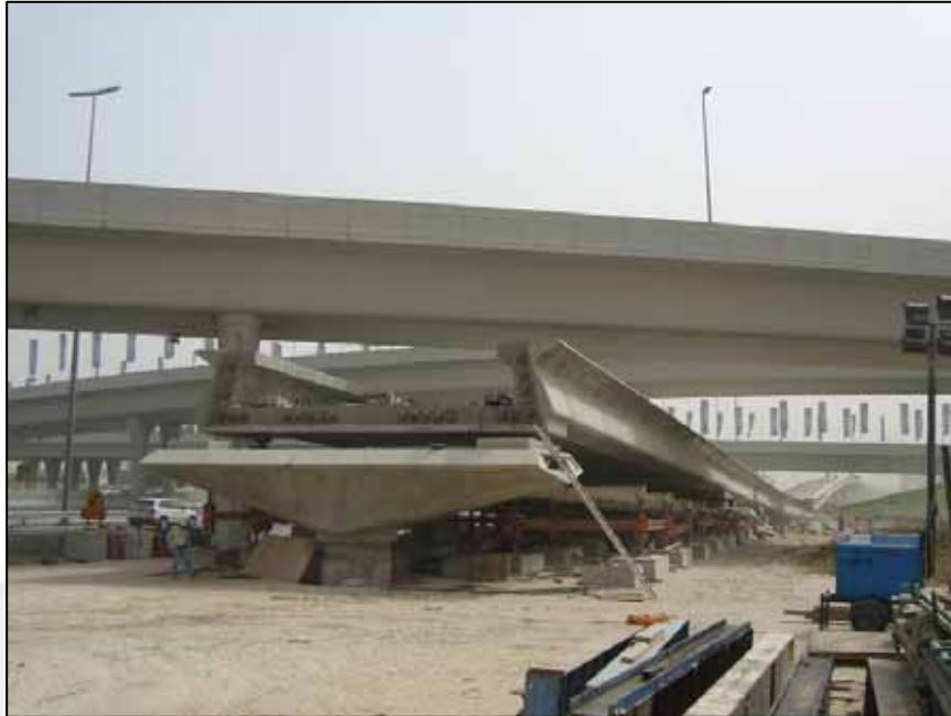
Existing road bridges at IC4.5
