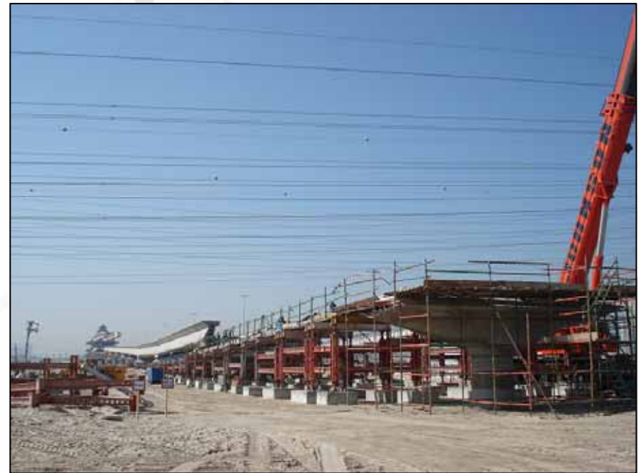
High voltage overhead power cables
