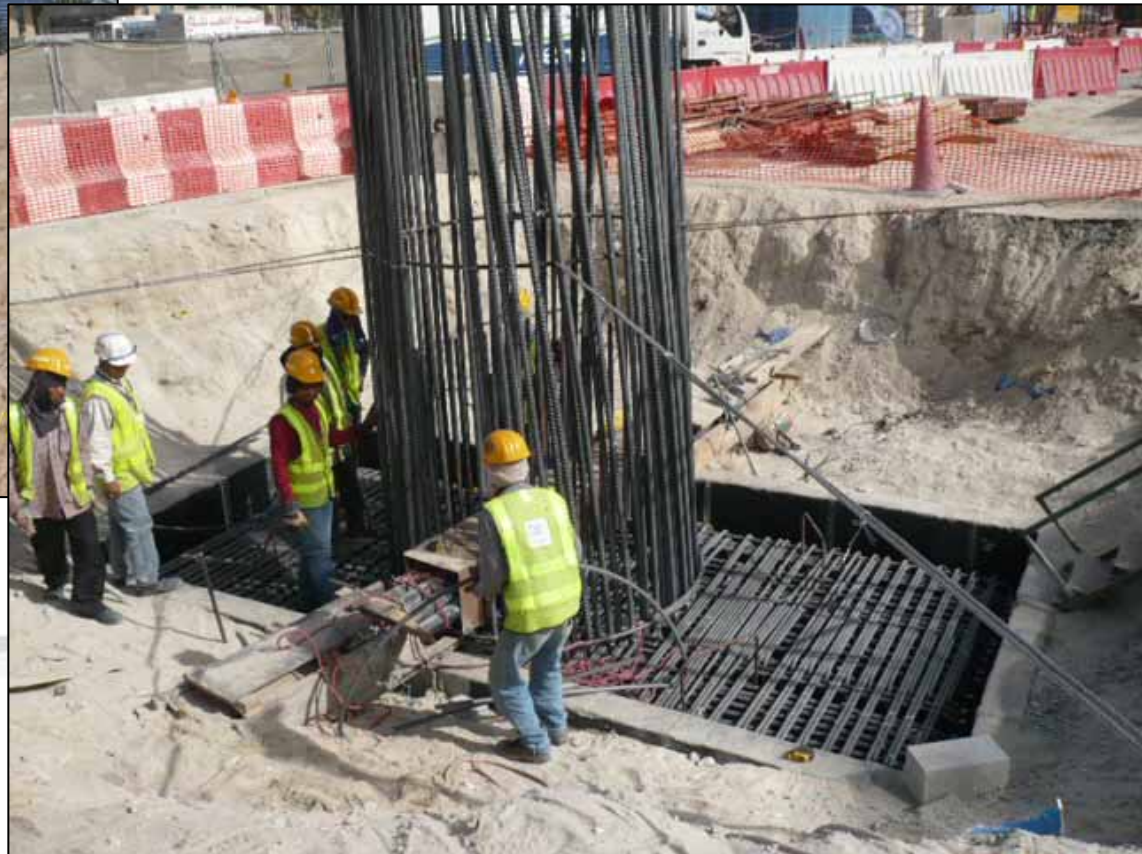
Etisalat cables through RPN325 Pier
