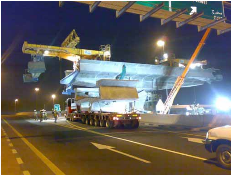
Work under complete road closure at Nadd Al Hammer
